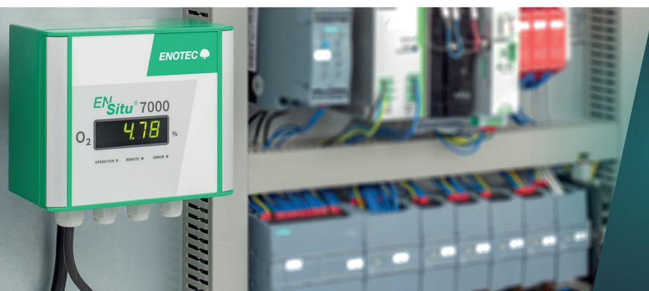
Designed for easy integration in existing boiler concepts. Detachable electronics for more convenient access.
